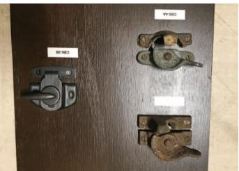
Samples of original hardware (top) facilitate restoration and, where necessary, replacement. Existing historical hardware may be removed and restored (right), then re-installed (bottom).
